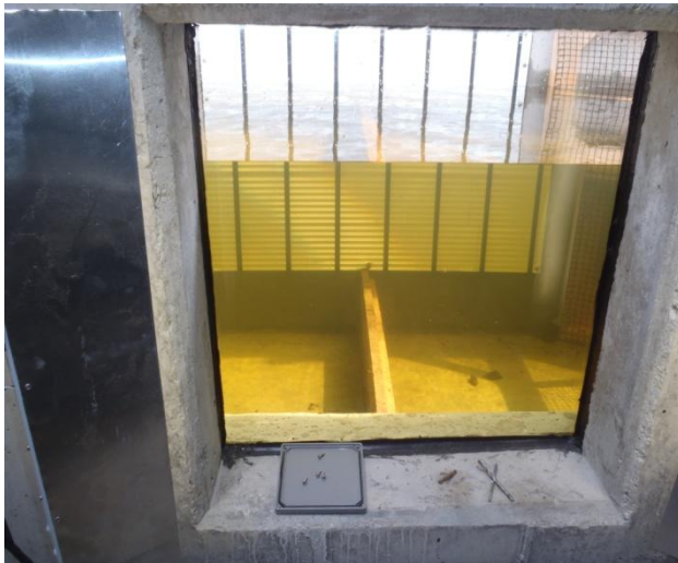
The viewing window at the new Hallville Fishway (Poquetanuck Brook, CT), which is now open and ready for business. The board on the bottom is a 'fish baffle' intended to keep fish from swimming below the window ledge and avoid detection. The backdrop is photo-reflective material to assist with low light images (with 6" stripes), and the mesh lead fence for the Smith-Root Electronic fish counter can be seen to the right. This fishway has both an electronic counter and a camera (for verification of species ID and direction of movement and public outreach).
