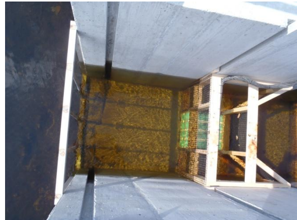
Top view of the Hallville Fishway exit (flow is from headpond, left to right). Trash rack is to left and the counting weir slides down a set of channels to the right just upstream of the viewing window. Fish are forced to swim through green PVC pipes to get counted. Cables go through formed portal in wall and enter the counting house where the instrumentation is housed along with the camera and computer for the imaging.
